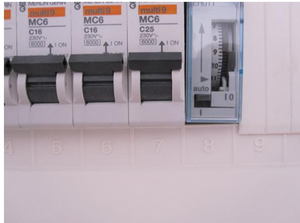
There is a water tank on the roof which holds 300 litres of water. When the water in the tank falls below 40 degrees and switch number 7 is on, the electric resistance in the tank kicks in and heats the water to 70 degrees. Having switch number 7 on at all times will ensure that the water never falls below a certain temperature. Heating 300 litres of water is likely to consume a lot of electricity so this may be an expensive alternative to ensuring there is always hot water when needed.
